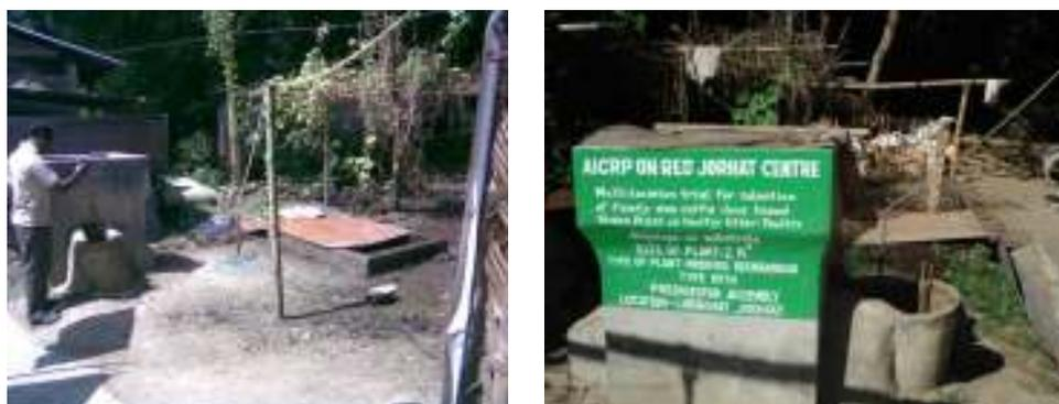
Figure (2): Side and front view of 2 m<sup>3</sup> plant with Pre-digester assembly.
